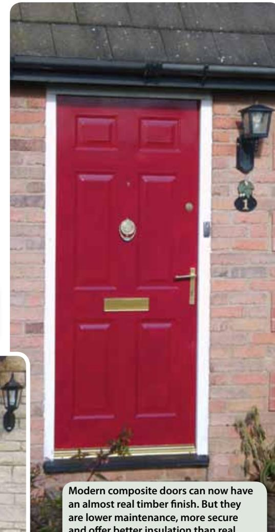
Modern composite doors can now have an almost real timber finish. But they are lower maintenance, more secure and offer better insulation than real wood. They have laminated subframes for added strength and a high-density, thermally efficient core that's comparable to the performance of insulation used in cavity walls.
