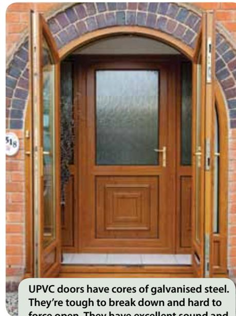
UPVC doors have cores of galvanised steel. They're tough to break down and hard to force open. They have excellent sound and heat insulation too.
